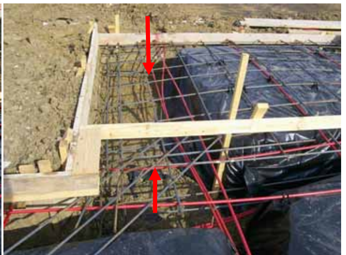
Recommend adding rebar in the lower footer.
