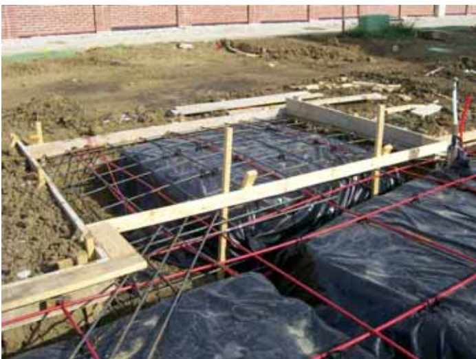
Recommend adding rebar in the lower footer.
