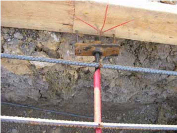
Cable ends need to be wrapped.
